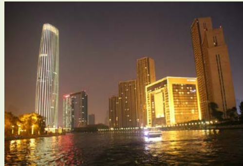
Tianjin 336.9m Jin Tower lighting project
